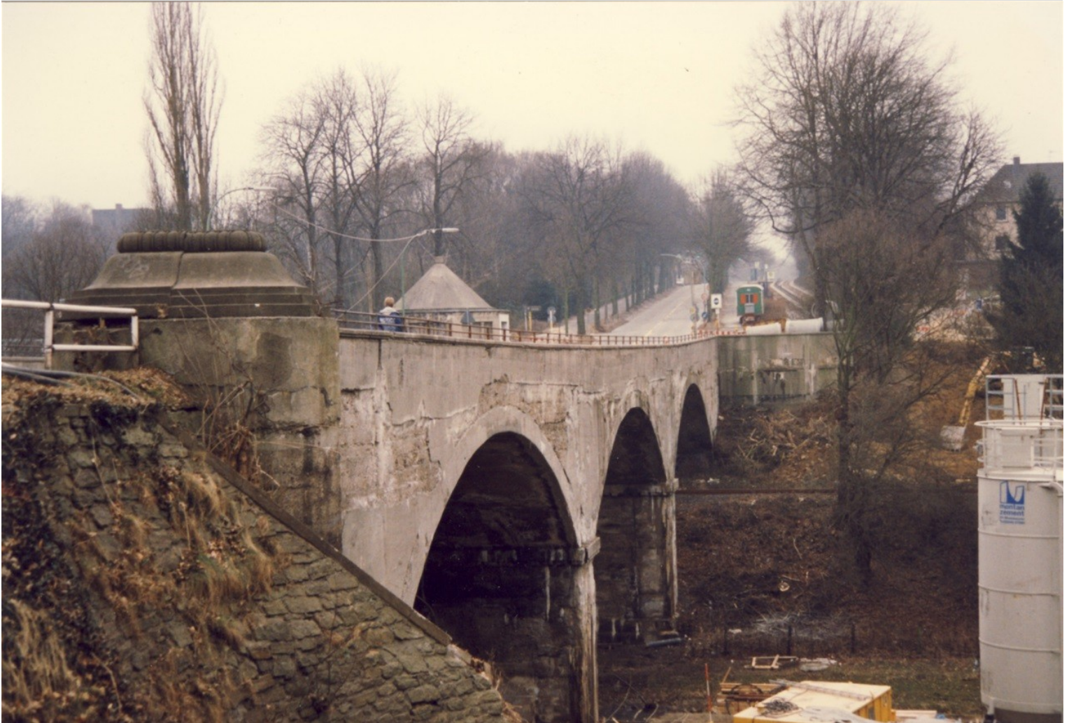
The original Wickenburgbrücke was torn down and replaced by the present one in about 1996. This view shows the western parapet of the old bridge. The demolition is already under way. In the distance: The trees of Southwest Cemetery where all Allied victims of that day were initially buried. (Photo: Sammlung Robert Welzel Essen)
